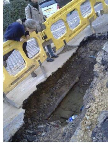
**On the left is a photo of a large cavity uncovered under Heath Street, outside the Baptist Church. To the right is a sink hole that appeared in New End. These illustrate the erosion of a significant volume of silt from the Claygate Beds by the action of groundwater, causing subsidence, cavities and sink holes. This action is magnified when basement developments constrain and thus speedup the groundwater flow.**
