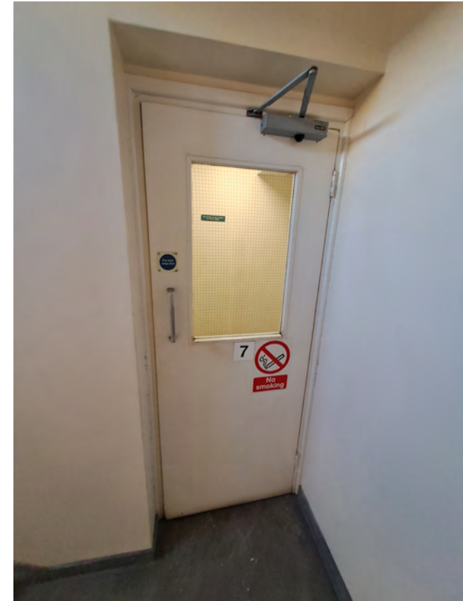
Communal Fire Door at 8 Newton Street
