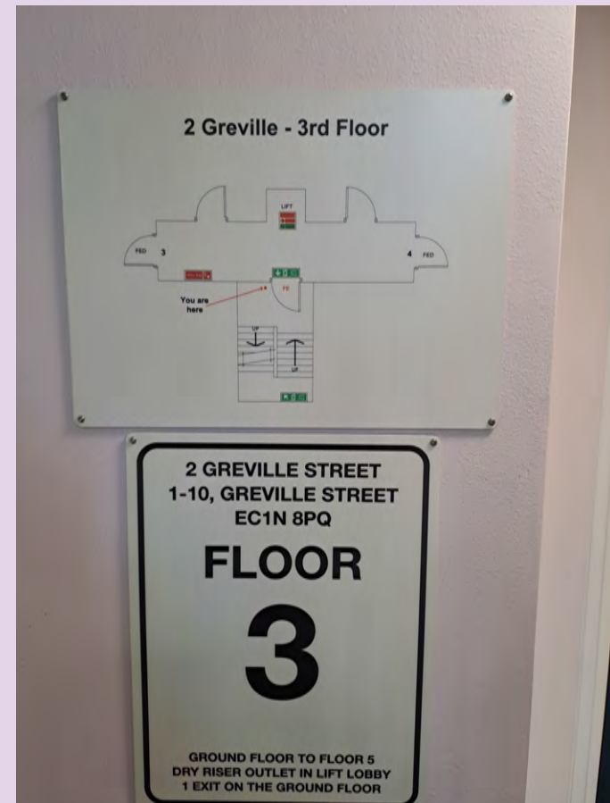
Wayfinding signage at 2 Greville Street.
