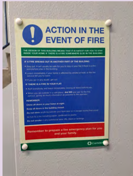
Fire Action Notice at 2 Greville Street.
