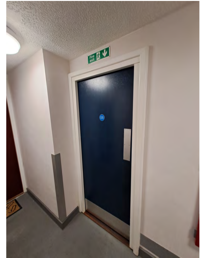
Fire door leading to stairwell at 2 Greville Street.
