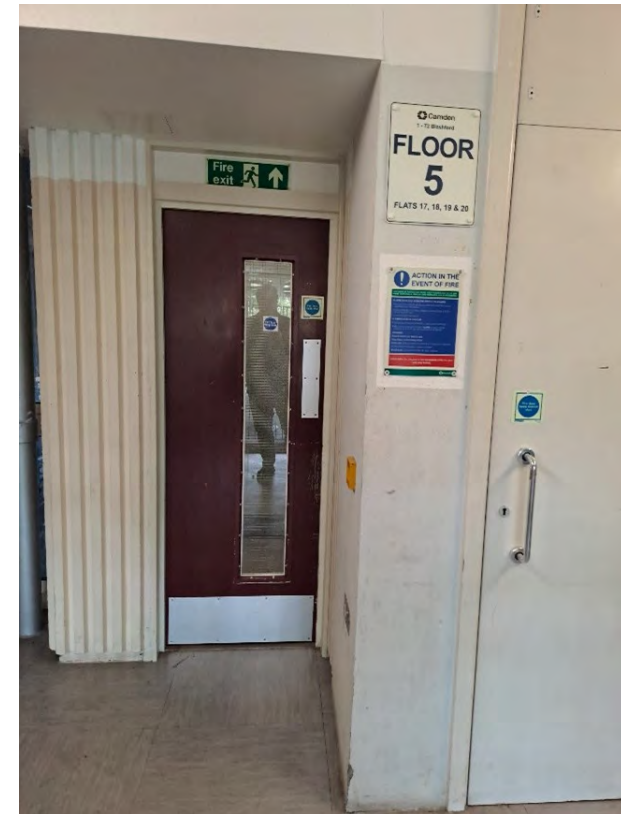
Communal area fire door at Blashford Tower.
