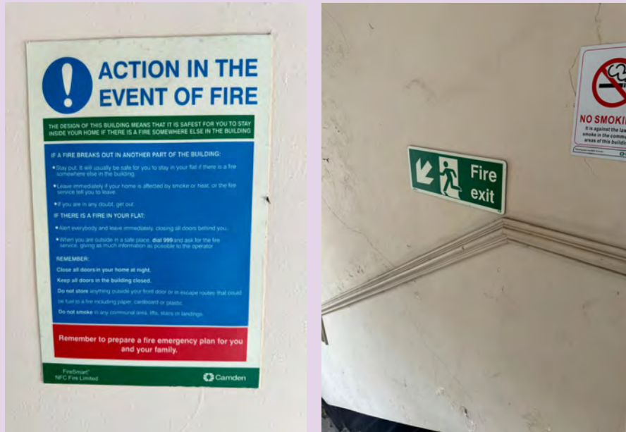
Fire Action Notice and Fire Exit Sign at Seymour House.
