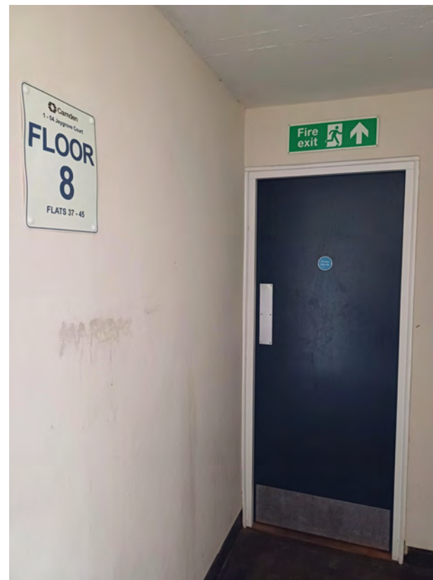
Communal Fire Door at 1-54 Jeygrove Court.
