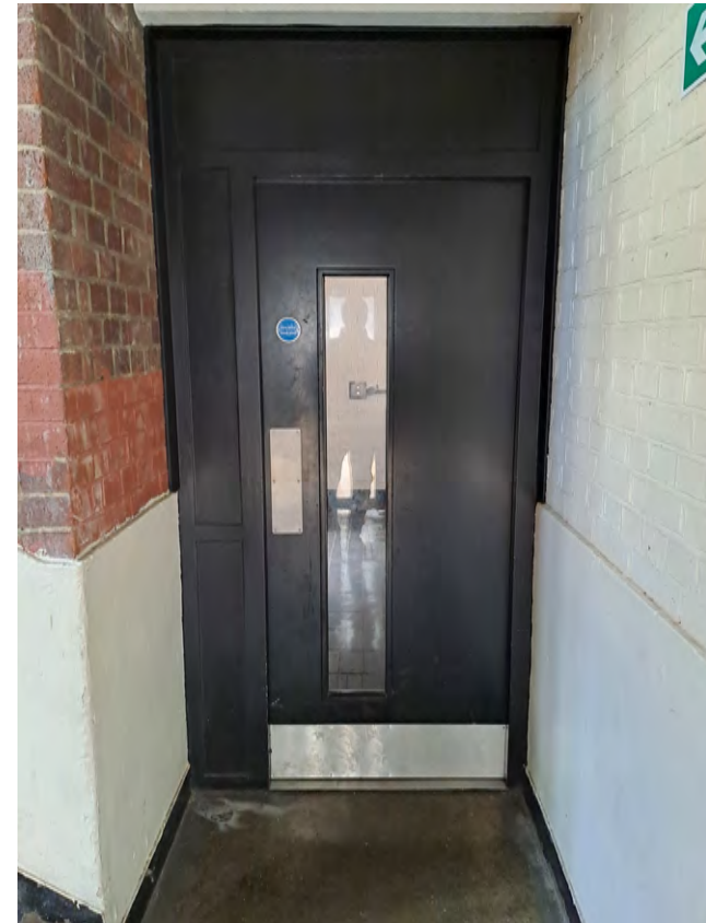
Communal area fire door at 1-35 Heybridge.
