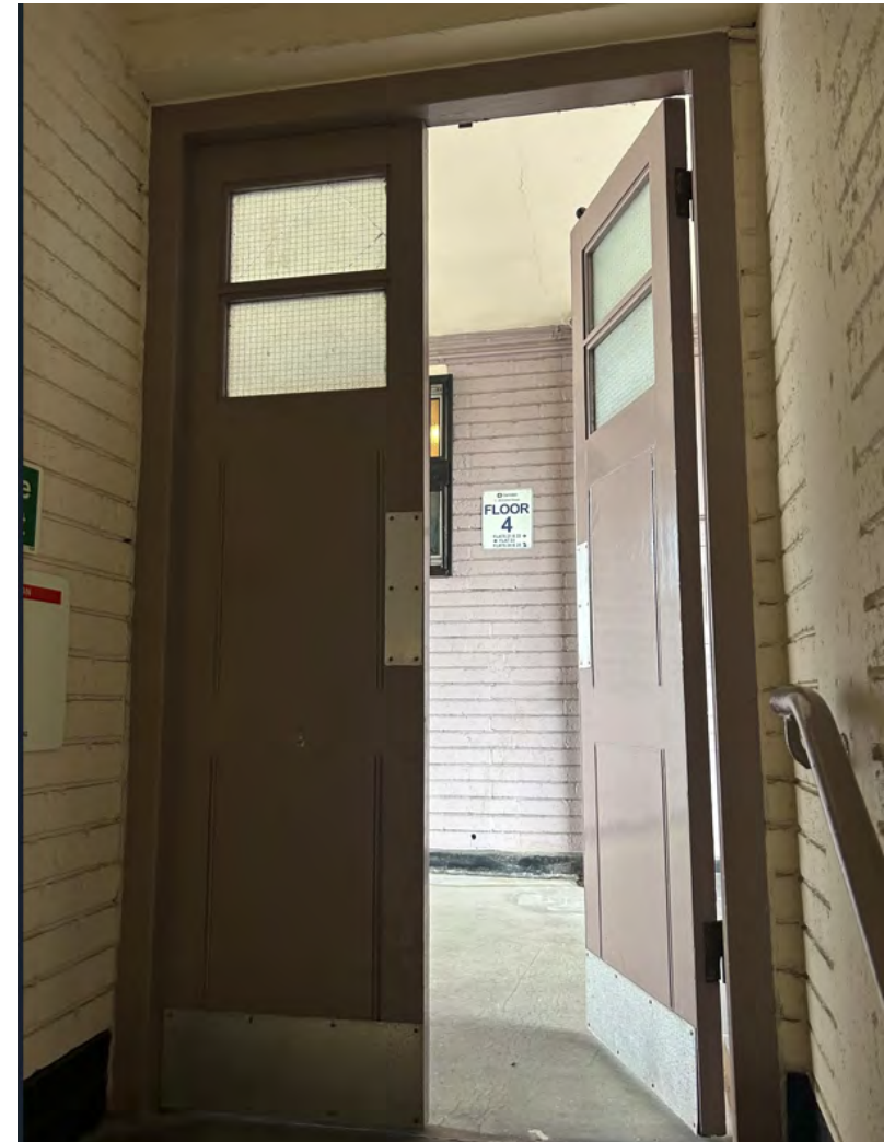
Communal Fire Door at 1-28 Culver House .
