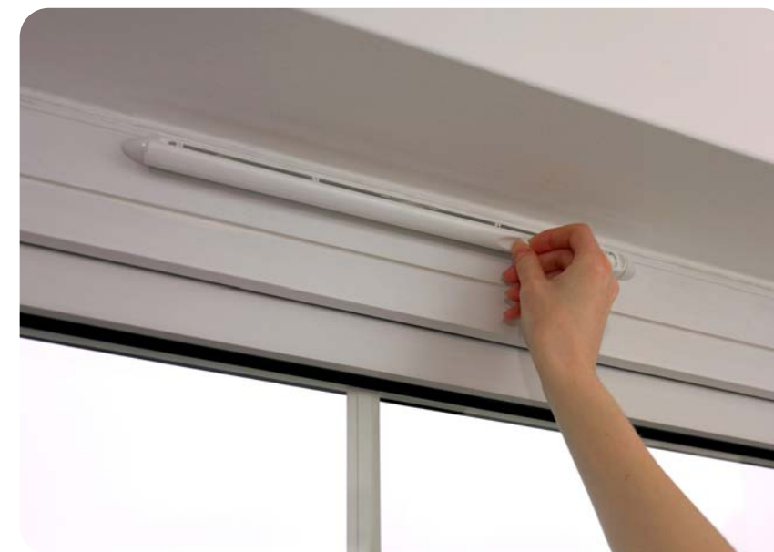
Example 2: Titon trickle vent
