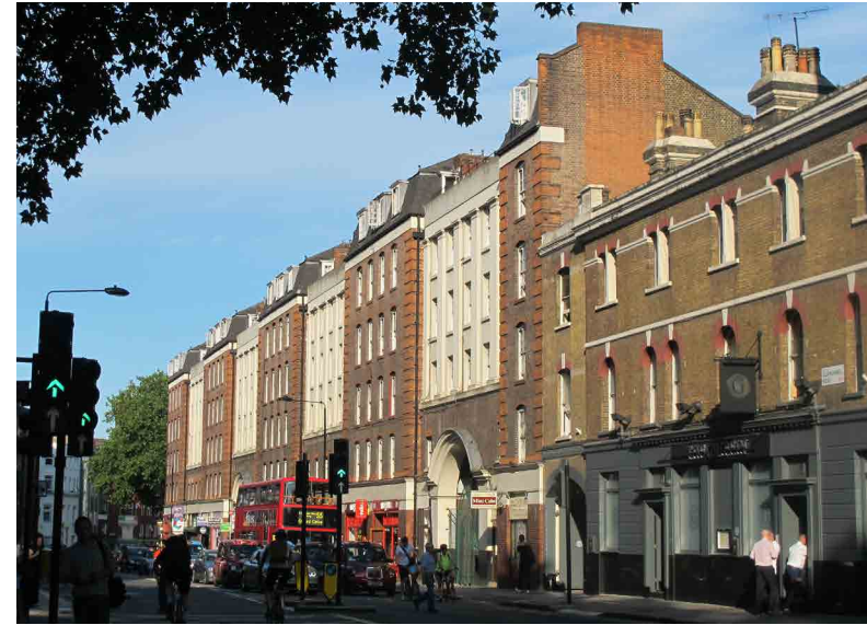
Bourne Estate, Clerkenwell Road frontage
