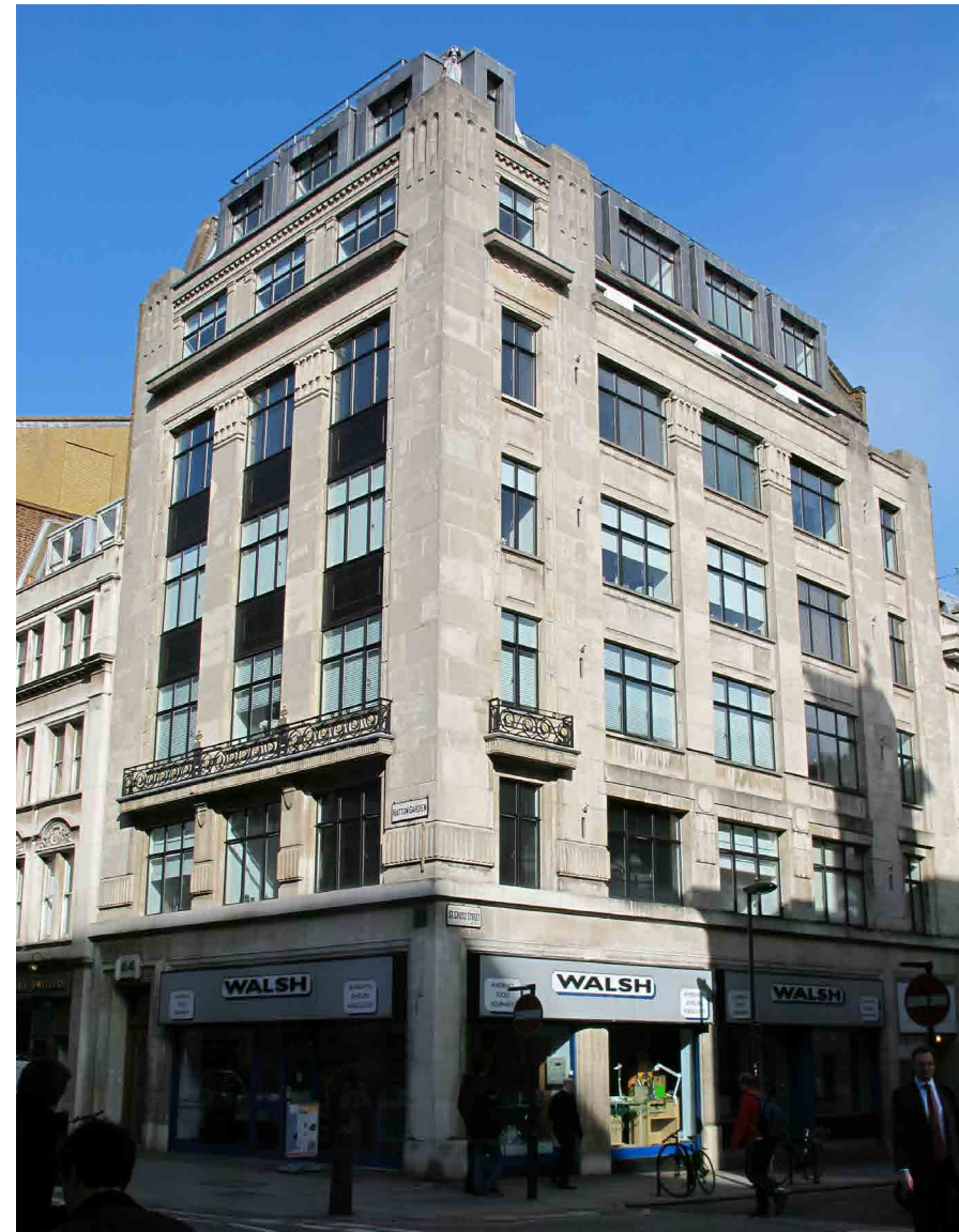
44 Hatton Garden: an Interwar commercial building, now apartments
