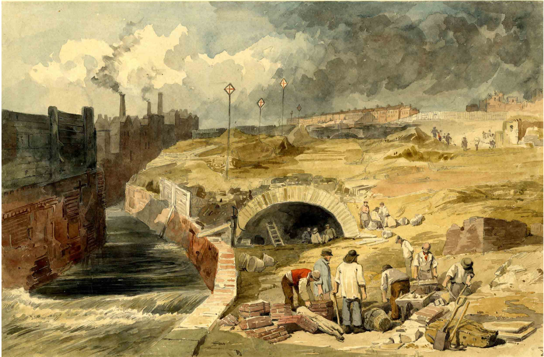
The site of Farringdon Road in 1855, showing the River Fleet (left) and the brick sewer being built to culvert it (right), following clearance of houses on Saffron Hill (watercolour by John Wykeham Archer, British Museum)
