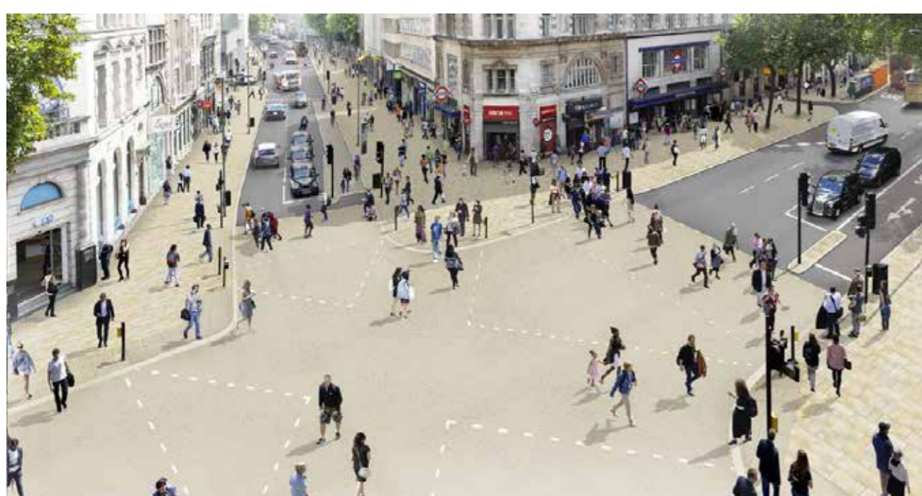
Pavement widening and new diagonal 'super crossing' currently being implemented as part of the Holborn safety scheme
