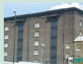
Part of the facade of the Granary
