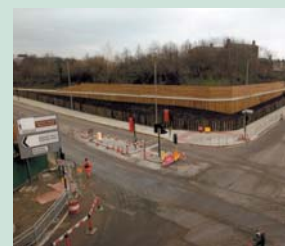
Camley Street Natural Park from station roof
