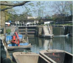
Canal, lock and dredger
