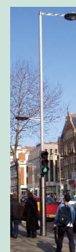
Carriageway lighting, footway lighting and signals mounted on a single column reduces street clutter
