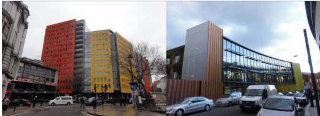
Figure 5.5: Examples of Large Office Provision (the St. Giles development in Tottenham Court Road and VIACOM Inc. building in Camden Town)
