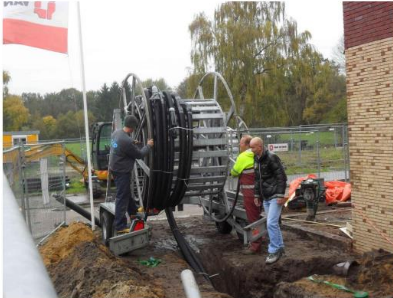
Figure 1: Preinsulated pipework
